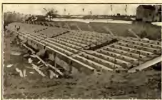
STADIUM UNDER CONSTRUCTION
