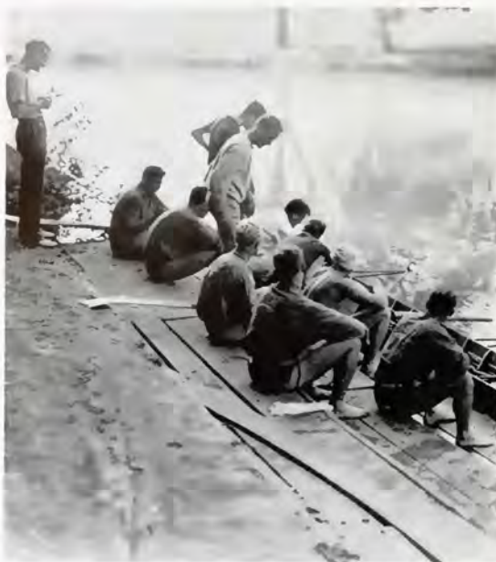
Rollins Crew relaxes between workouts on North River
