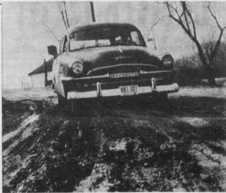
A temporary improvement has been made since this picture was taken at Hillside Terrace Wednesday, but unless this roadway is oiled the same condition will exist in a few weeks. —Aukschun photo.
