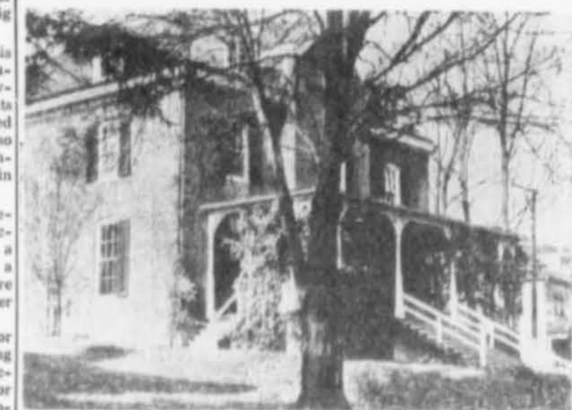
POTENTIAL ALUMNI HOUSE used to be the home of the late Dr. Fitzgerald Flournoy, former Professor of English at Washington and Lee. The Alumni Board will consider the Flournoy House at a meeting to be held during Parents' Weekend, according to Alumni Executive Secretary William Washburn. Several alumni committees approved the home for an Alumni House. The Lynchburg firm of Clark, Nelson and Owen submitted the plans for the renovation of the Flournoy home. Washburn emphasized that all aspects of the use of Dr. Flournoy's home are in the investigative stage.
