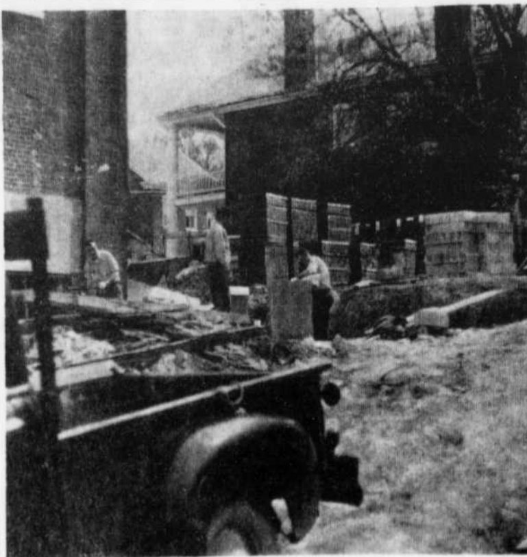
Lobby construction well under way.
