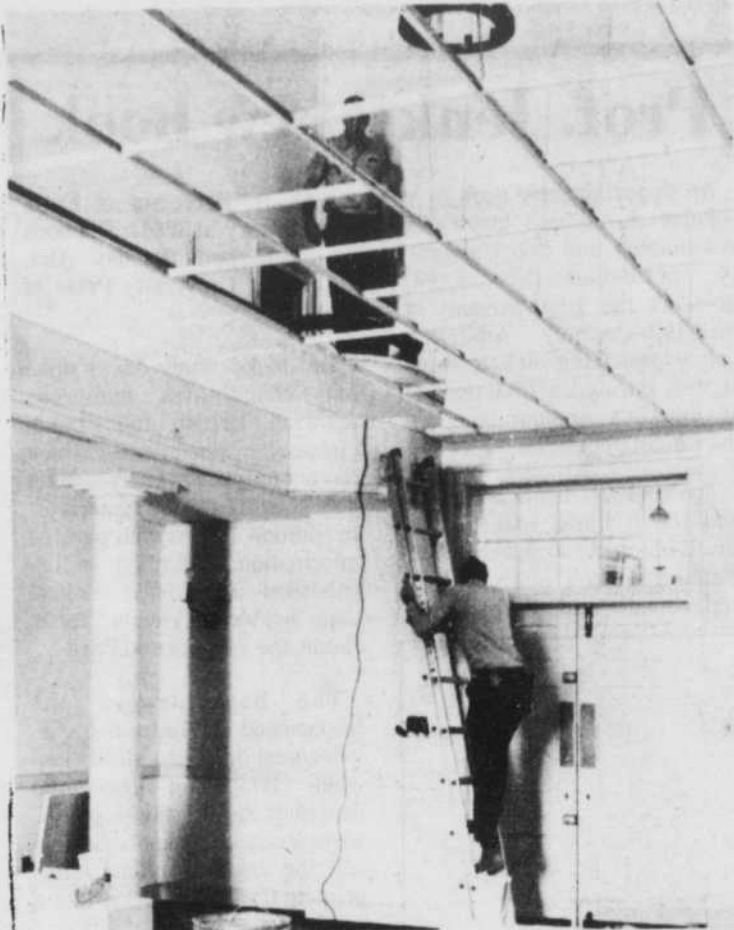
Enjoy your last glance at the classical-high ceilings in the admissions office; progress has even hit these hallowed halls as workmen install a modern lighting system.
