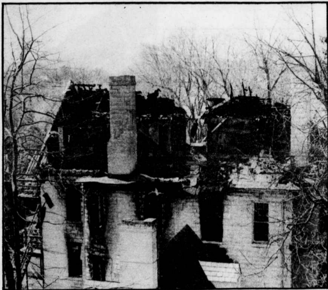
An aerial view shows the wreckage an early morning fire caused at the Phi Gamma Delta house. All three floors collapsed into the basement. More photos on pages 2 and 3. (Photo by Rick Swagler)
