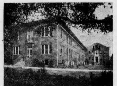
One of the three wings of the Jackson Laboratory, where a large portion of the basic research on dyes is carried on. The new $1,000,000 addition on the right is nearing completion.
