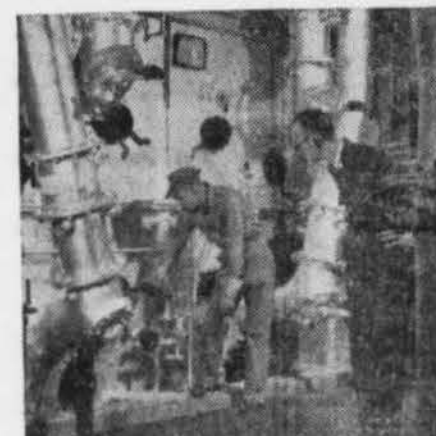
A FIREMAN adjusts a valve for the proper combustion of pulverized coal. Blown into furnace through pipes, it burns at 2500°F.
