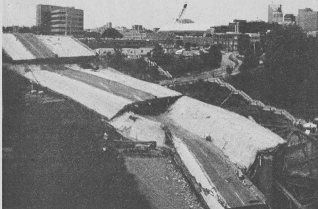
What remained of the I-35W Mississippi River Bridge in Minneapolis after it collapsed in 2007. The collapse could have been prevented by Peckens' biologically-inspired sensing nodes.
