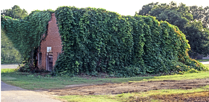
Blighted Building Swallowed by Kudzu in Helena, Arkansas
