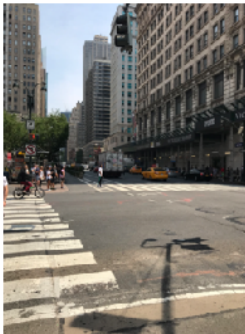
Figure 4: Scaffolding on Sixth Avenue to the right of Herald Square
