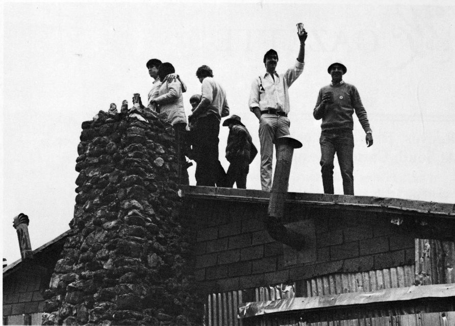
Rooftop revelers at Zollman's.
