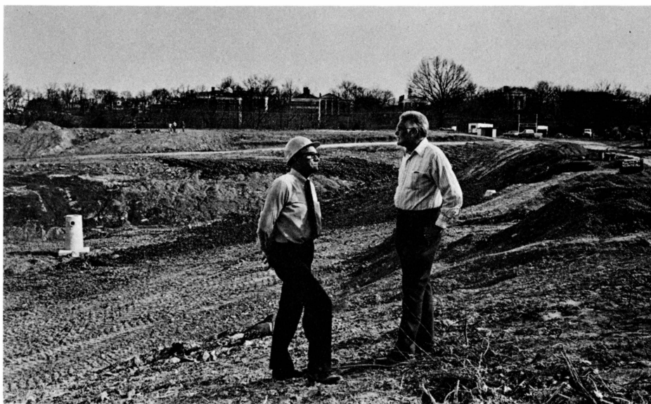
Projects Manager Pat Brady and Mack Parsons, representative of Kane construction company, inspect site of law school building.
