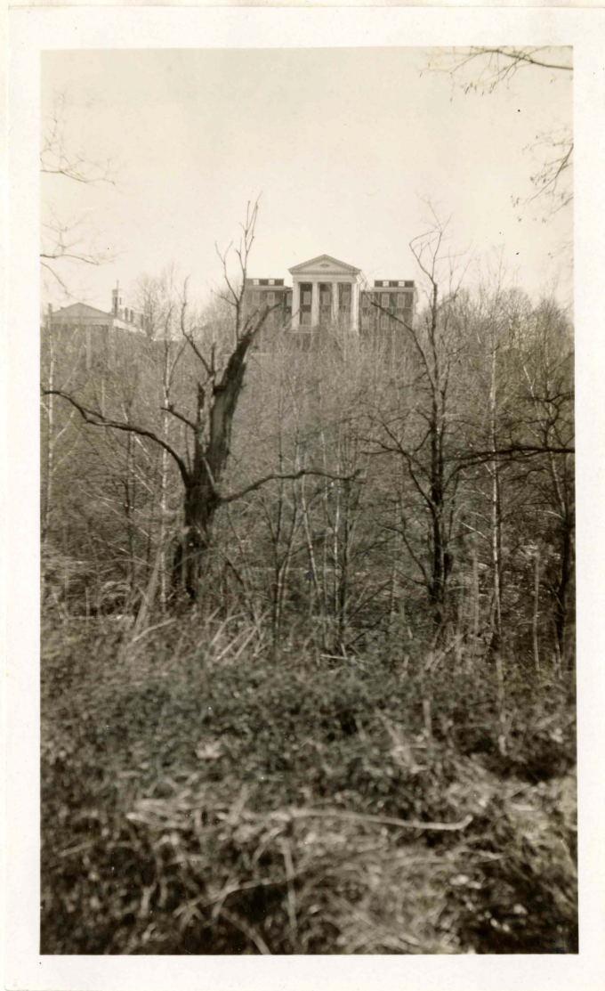
LOOKING ACROSS THE RAVINE FROM A POINT ON THE B. & O. R. R., SHOWING PART OF SITE OF PROPOSED LAKE
