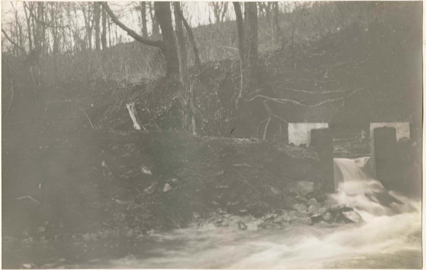
VIEW OF WEIR DAM
