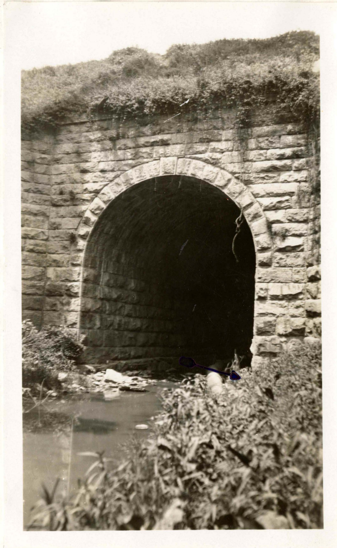
VIEW OF CULVERT SHOWING LOCATION OF BENCH MARK AS INDICATED
