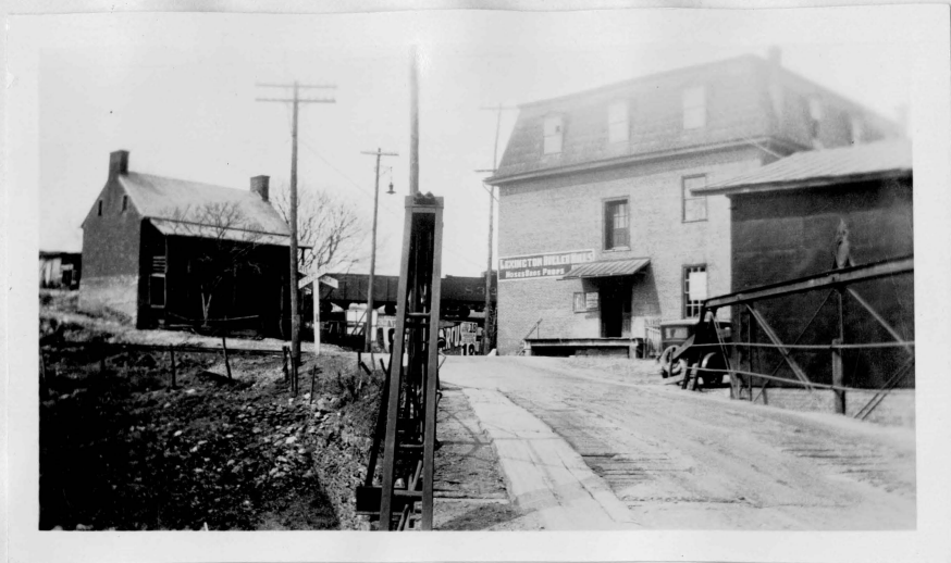
Curve at Moses' Mill Showing present pony truss
