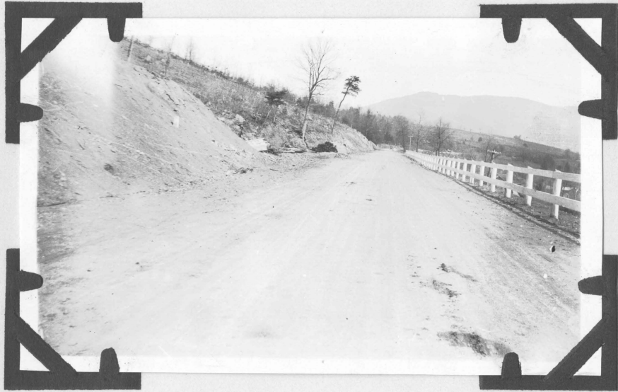
Completed stretch of macadam road. Including grading, drainage, surface, dressed shoulders, guard rail, and right of way monuments.
