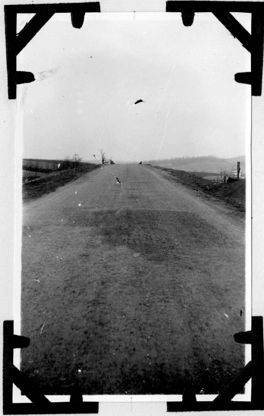
Good surrace on deep fill.
