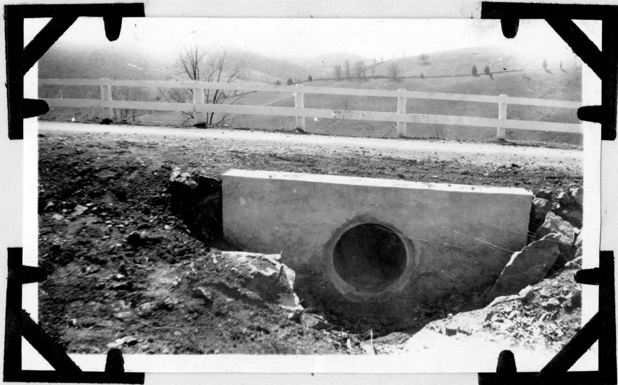
Headwall conforming to grade.
