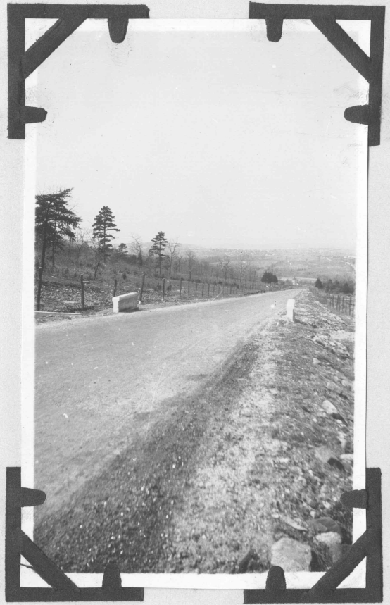
Box culvert handrails not conforming to grade.
