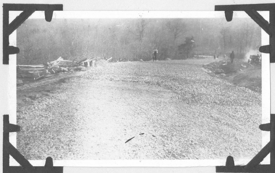
Number two stone ready to penetrate.
