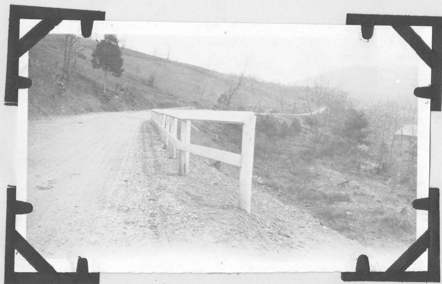
Winding mountain road; old type wood guard rail.
