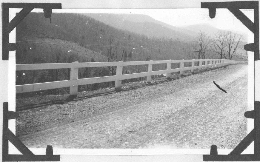
Completed wood guard rail.
