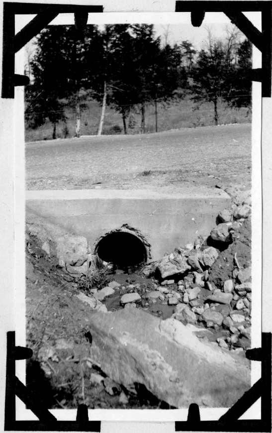
Headwall not conforming to grade.
