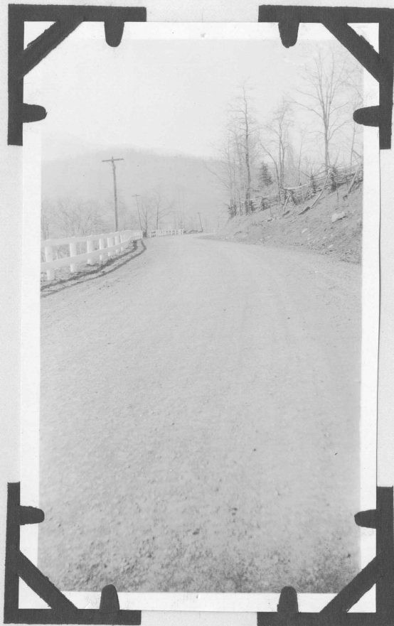
Completed section of mountain road.
