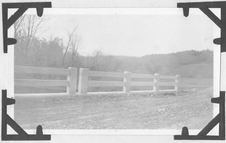
Concrete bridges; showing old and new type handrails.
