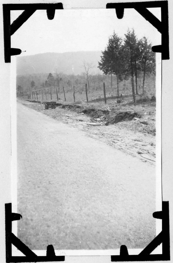
Headwall not conforming to grade.
