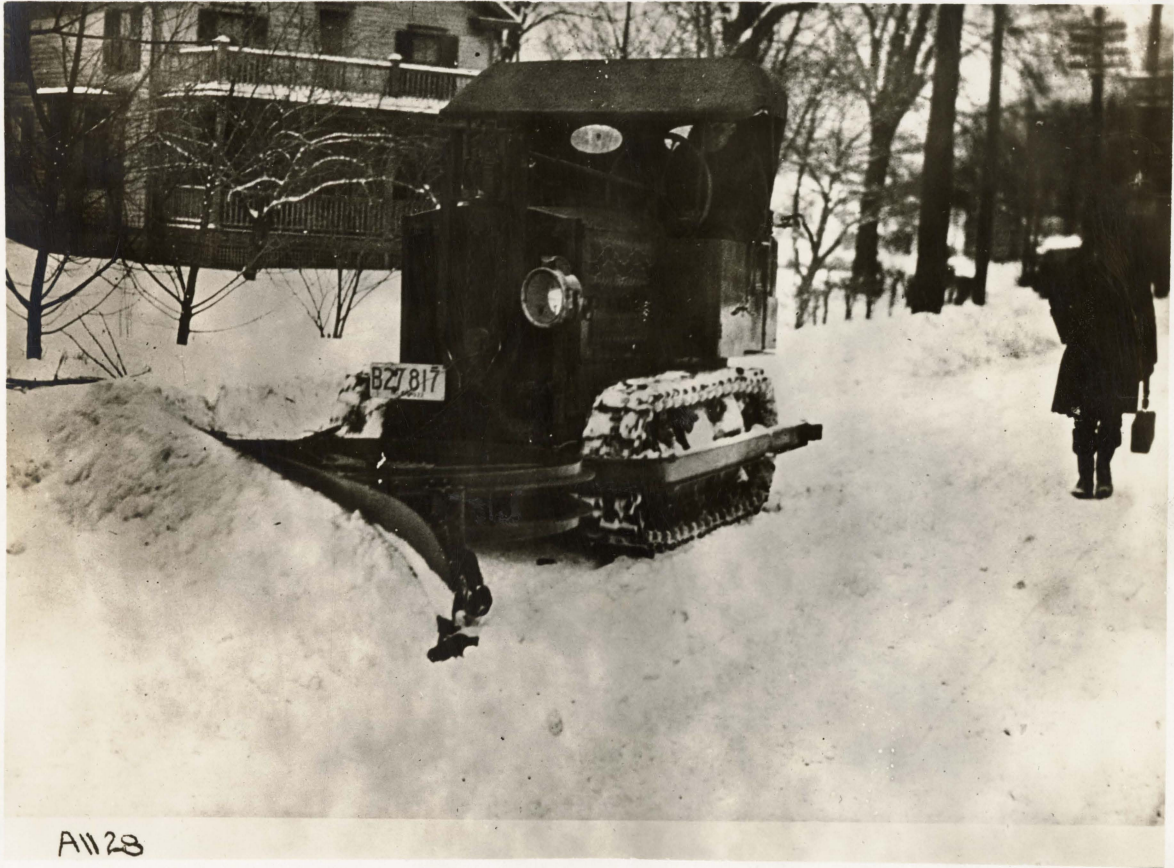
SNOW PLOW ATTACHMENT ON CRAWLER TRACTOR
