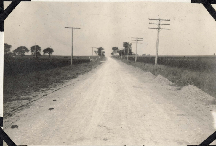
CHIPS PILED ALONG ROADWAY
