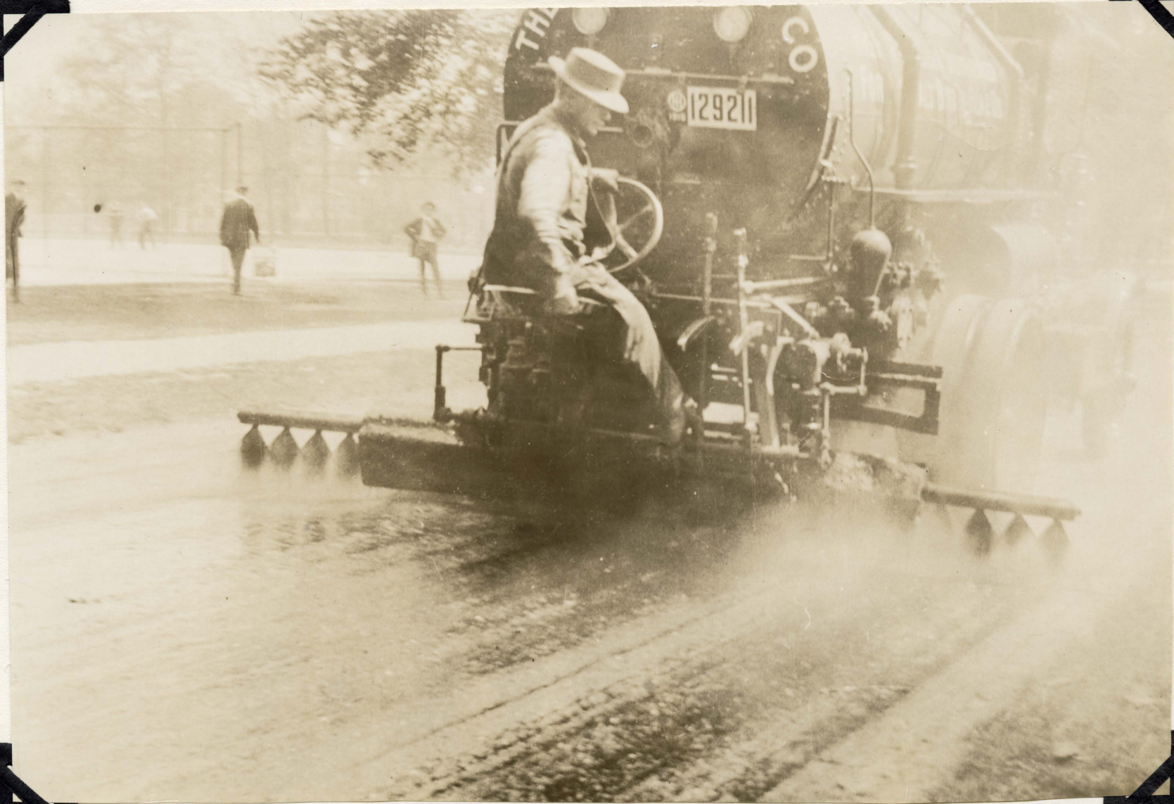
APPLYING BITUMINOUS MATERIAL TO A GRAVEL ROAD
