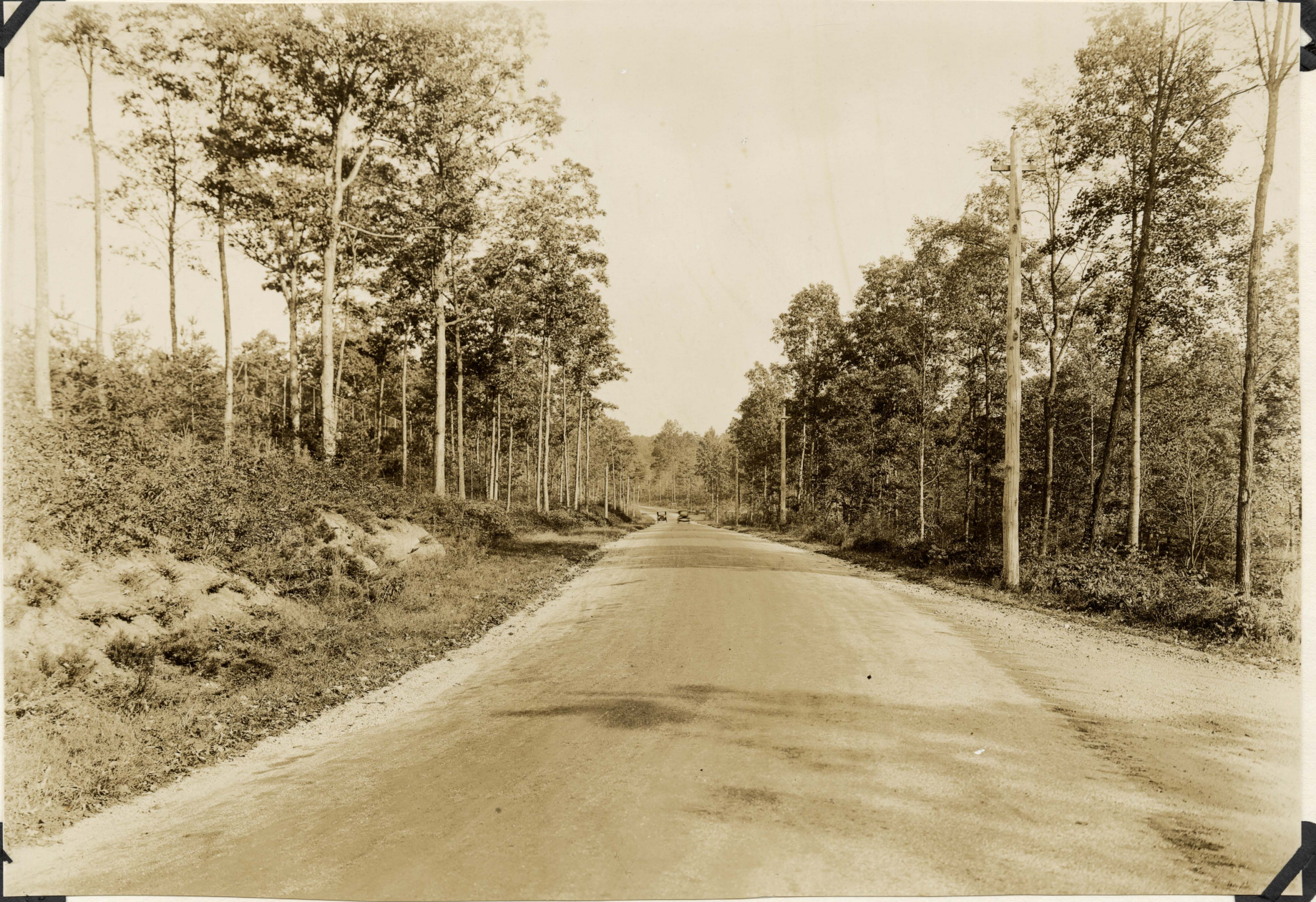
SURFACE TREATMENT COMPLETED
