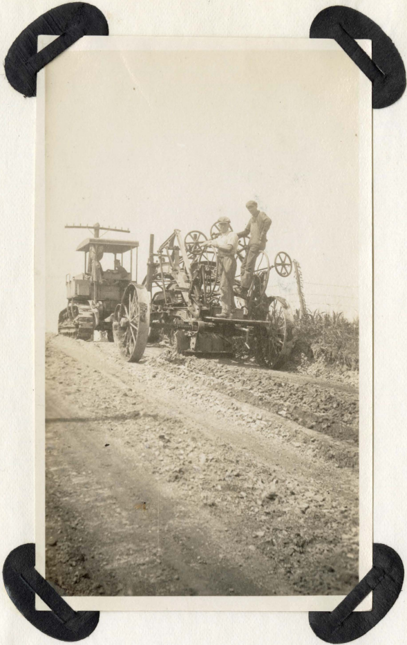
SHAPING A SHALE ROAD
