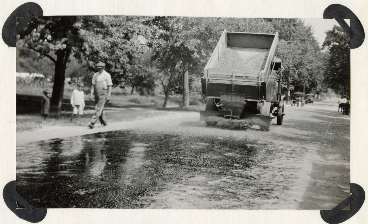
MODERN EQUIPMENT FOR LOADING STONE CHIPS AND COVERING BITUMINOUS TREATMENTS
