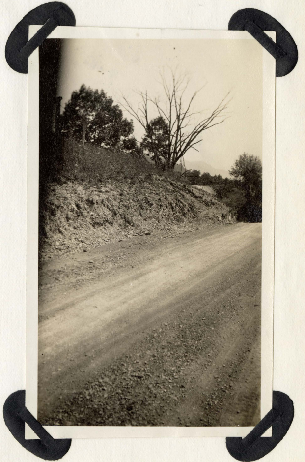
SAME ROAD AFTER IT HAS WORN SMOOTH UNDER TRAFFIC
