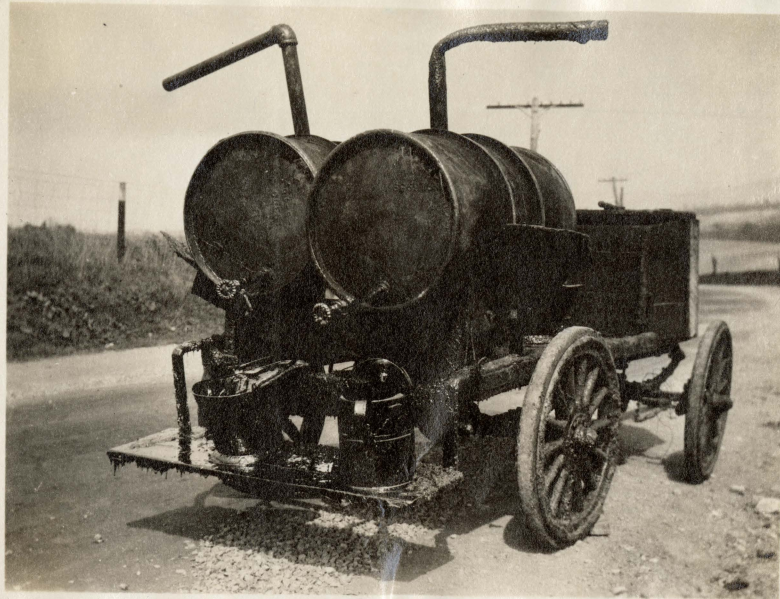
ARRANGEMENT FOR HEATING PATCH MATERIAL
