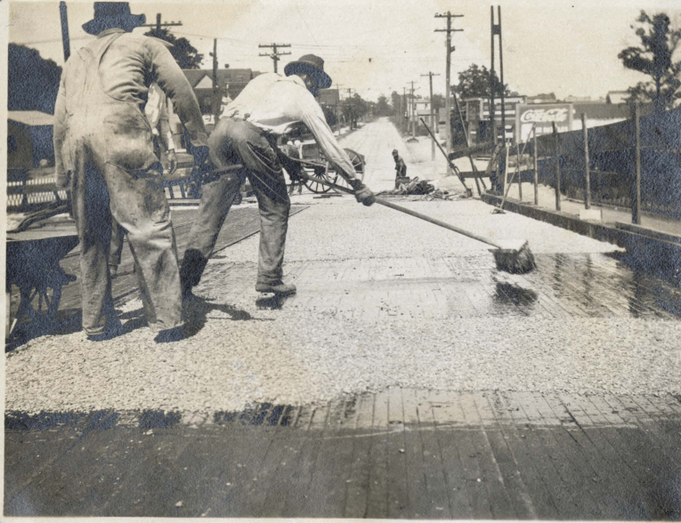
SURFACE TREATING A BRIDGE FLOOR
