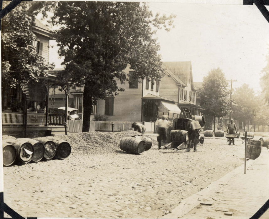
PREPARING COBBLE STONE FOR BITUMINOUS TREATMENT
