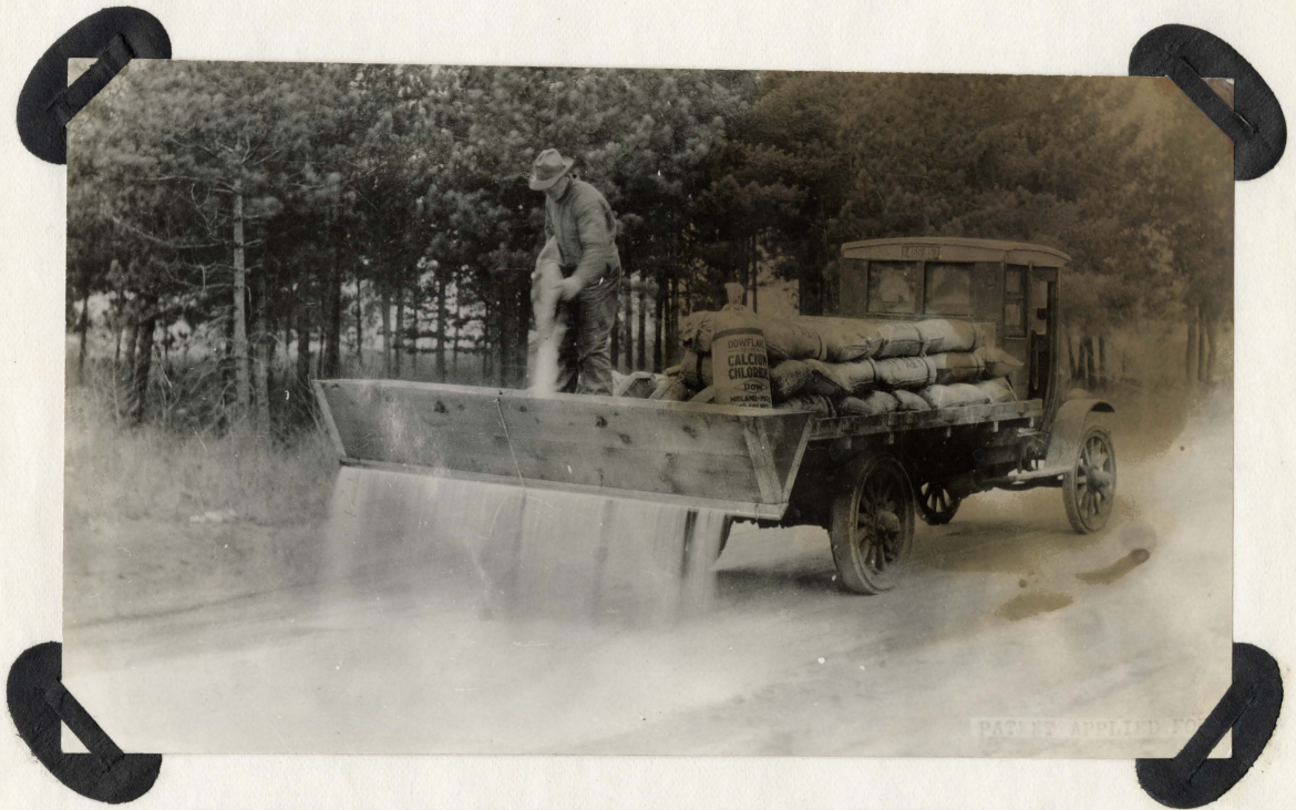
APPLYING CALCIUM CHLORIDE TO AN EARTH ROAD
