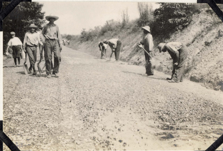
SPREADING CHIPS BY HAND
