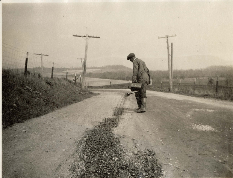
SPREADING PATCH MATERIAL
