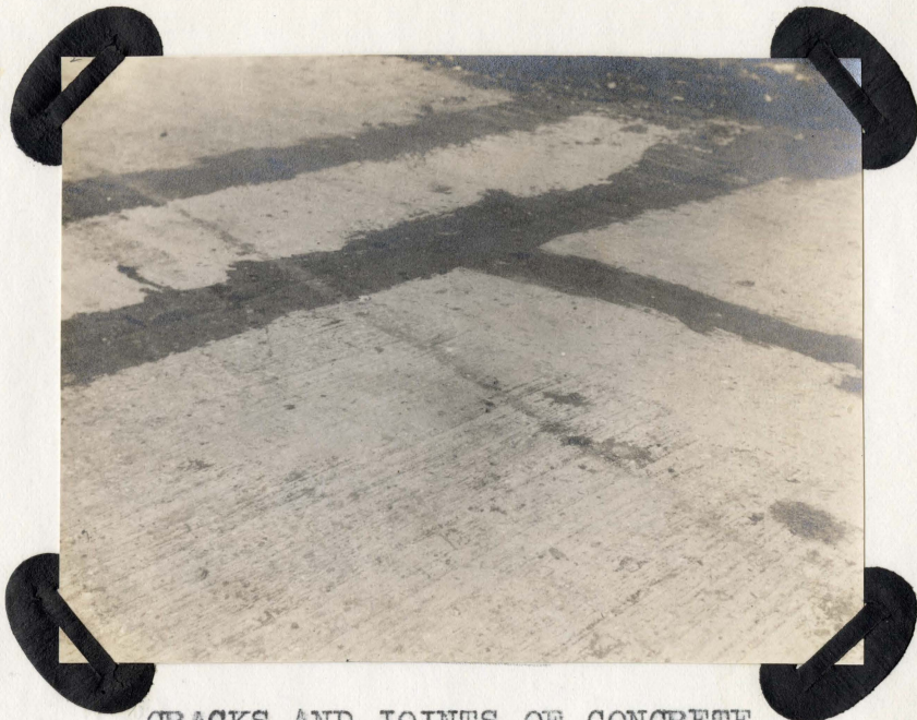
CRACKS AND JOINTS OF CONCRETE PAVEMENT FILLED WITH BITUMEN
