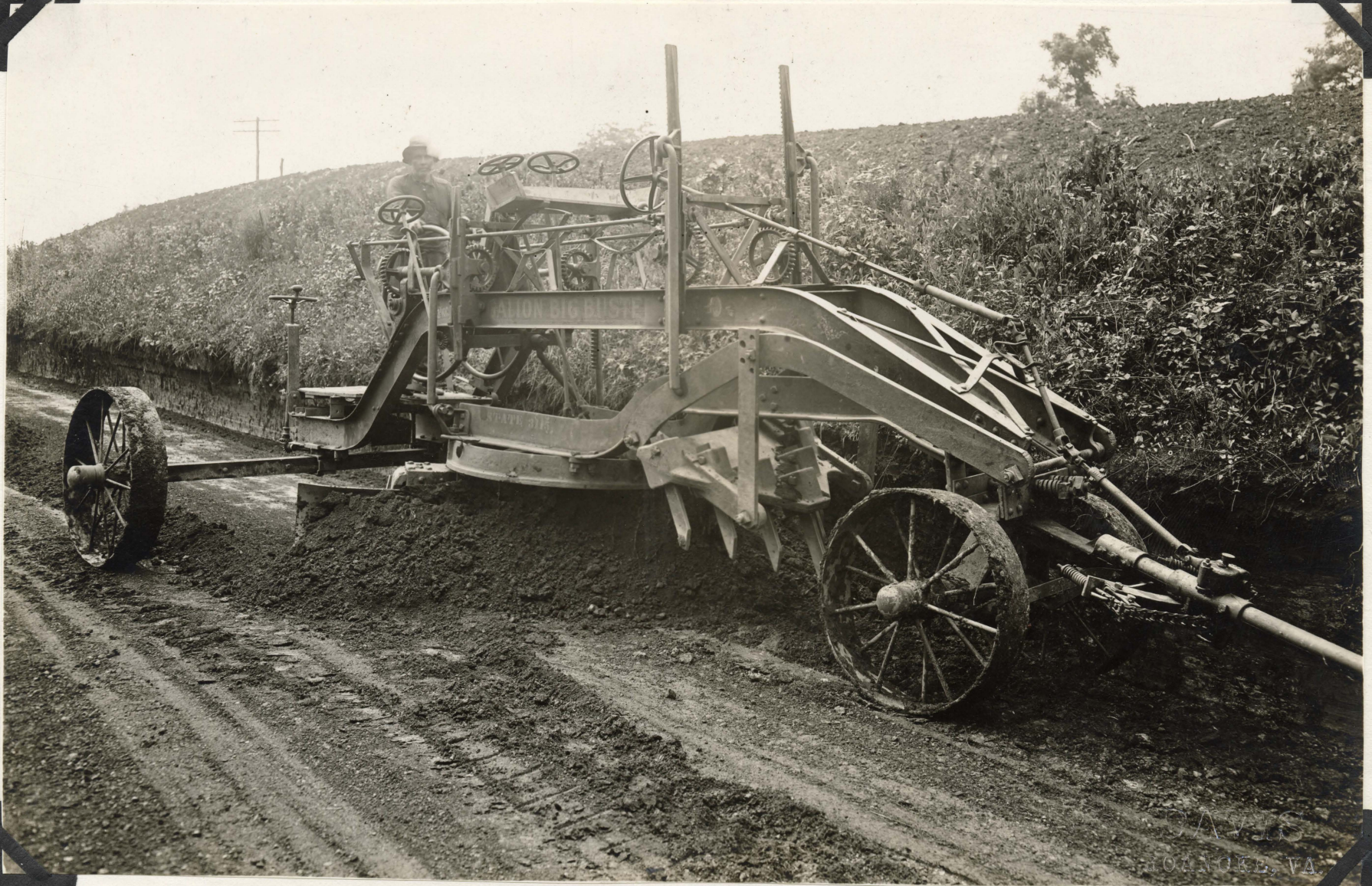
LARGE ROAD GRADER WIDENING ROADWAY
