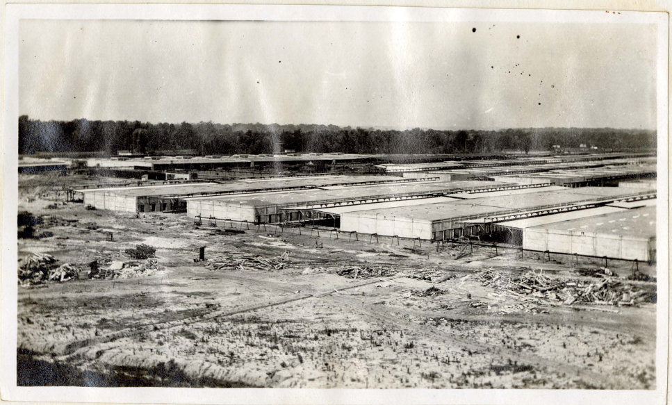
Some completed warehouses.
