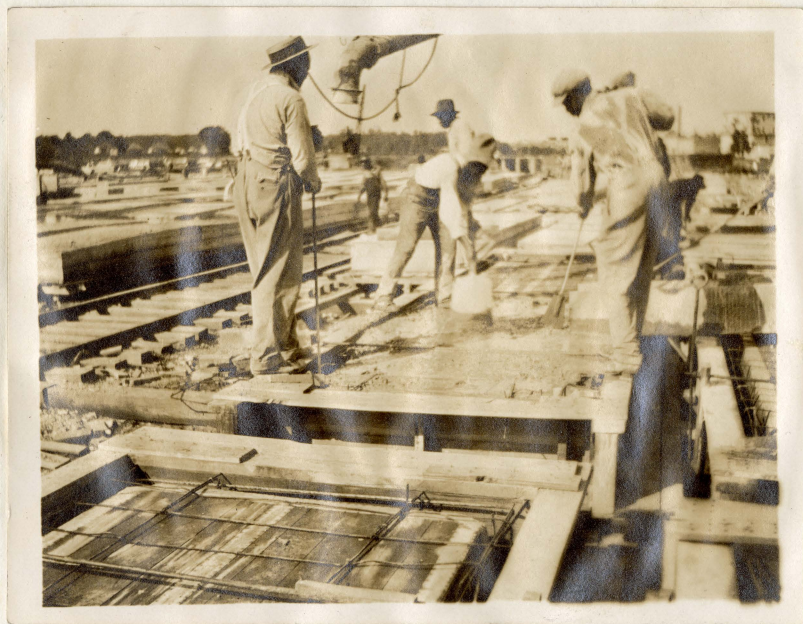
Pouring roof slabs. Note empty form.
