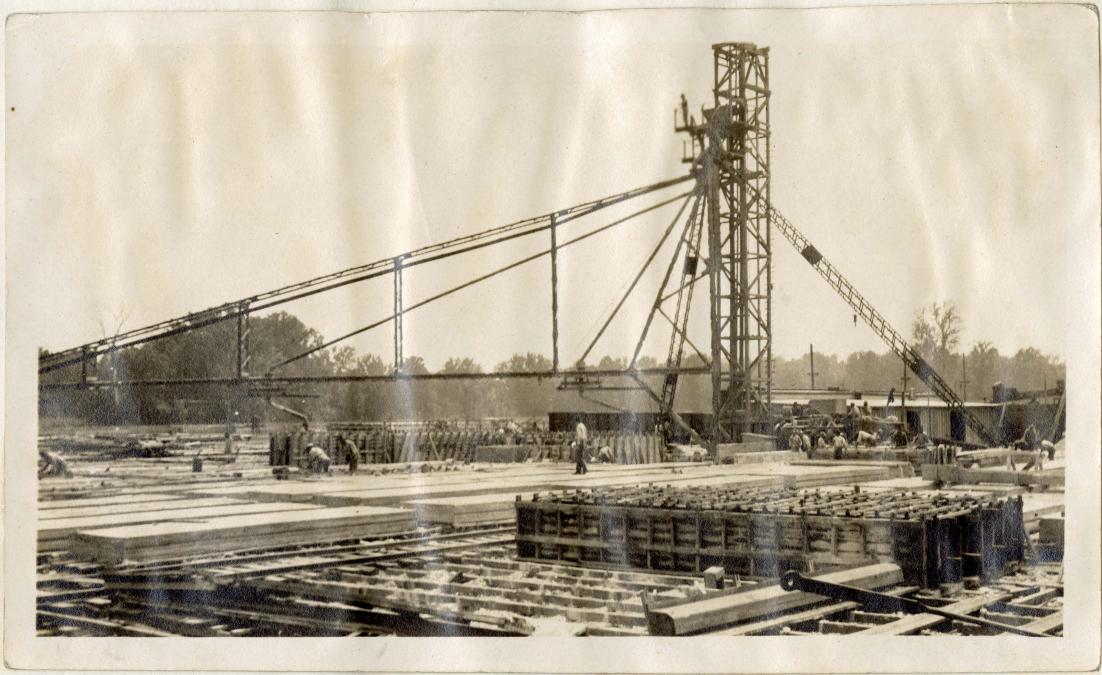
Casting yard and distributor.
