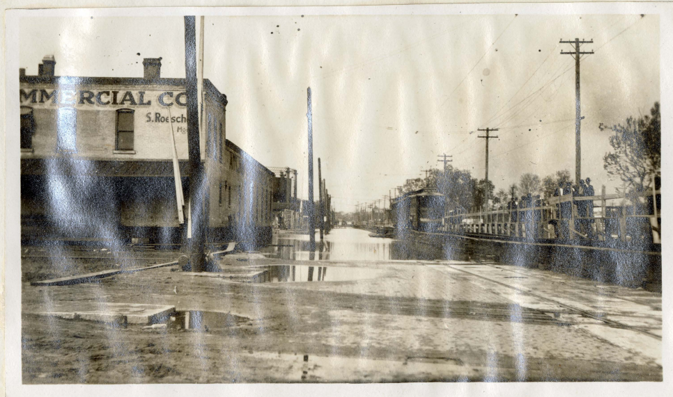
Overflow. Note elevated car tracks and walkway.
