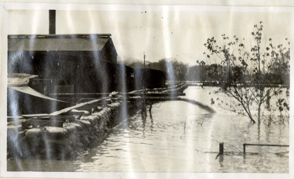
Industrial plant with sand bag levee. Note Seepage pumps.
