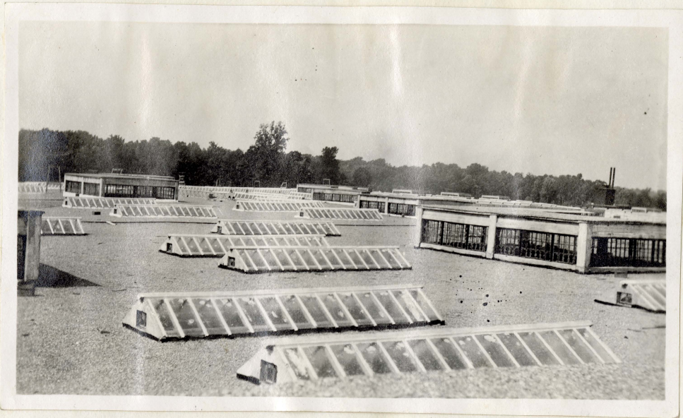
View of a roof. Note concrete ribs in sky light.
